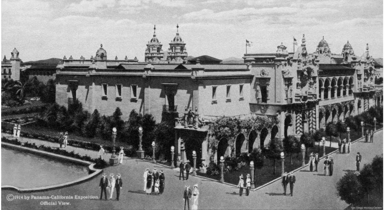
Varied Industries Building, San Diego Panama-California Exposition.
